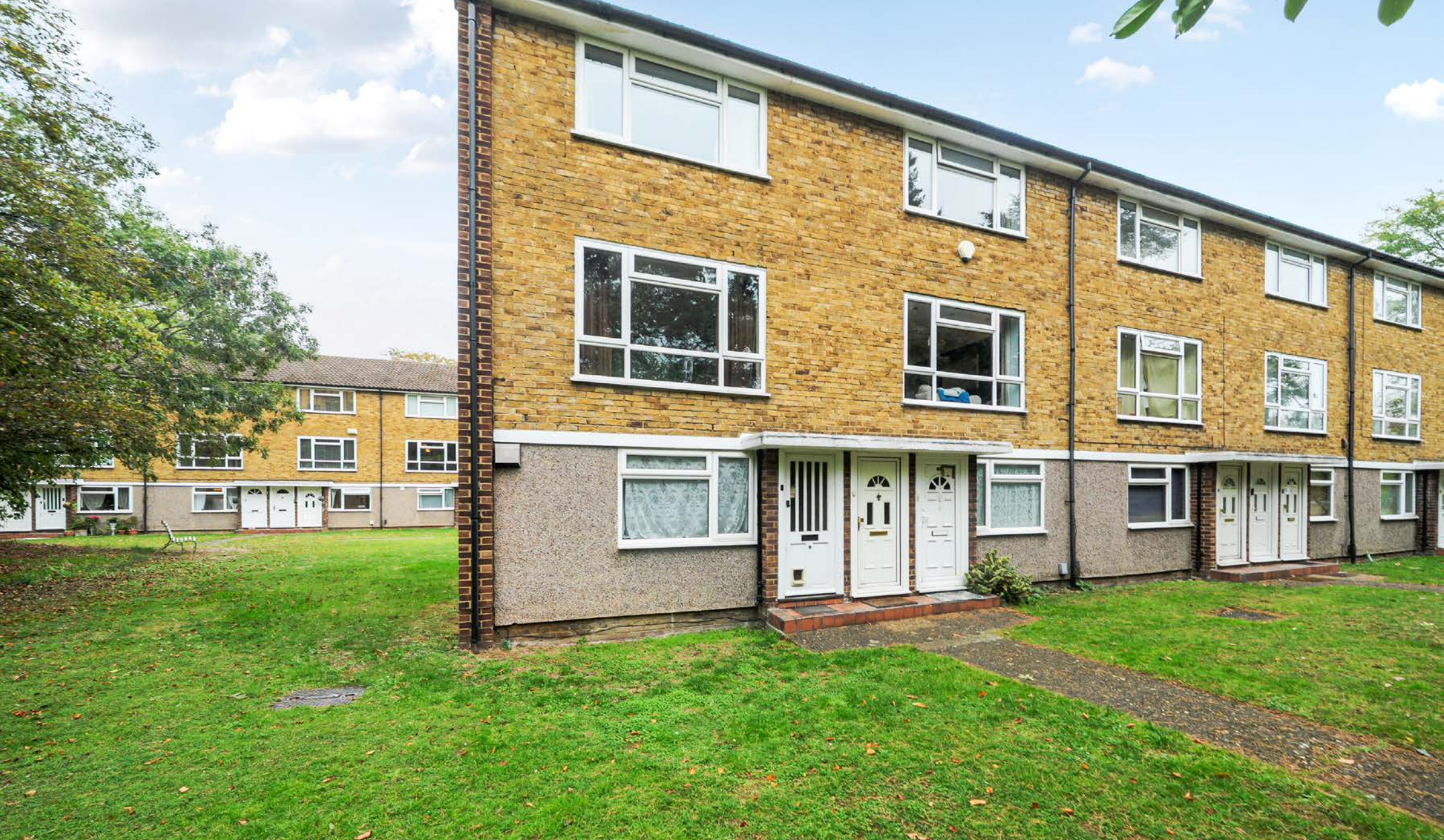
BEECHES COURT, AVONDALE ROAD BROMLEY, BR1
