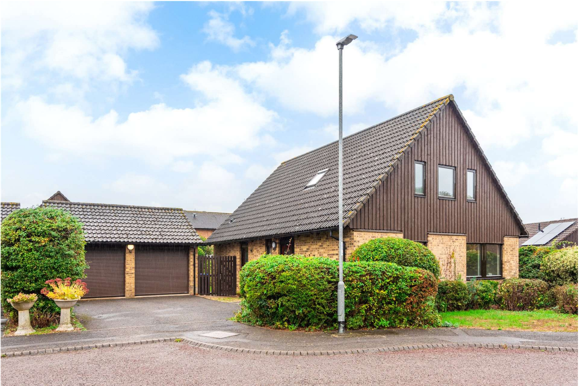
West Hunsbury, Northamptonshire
