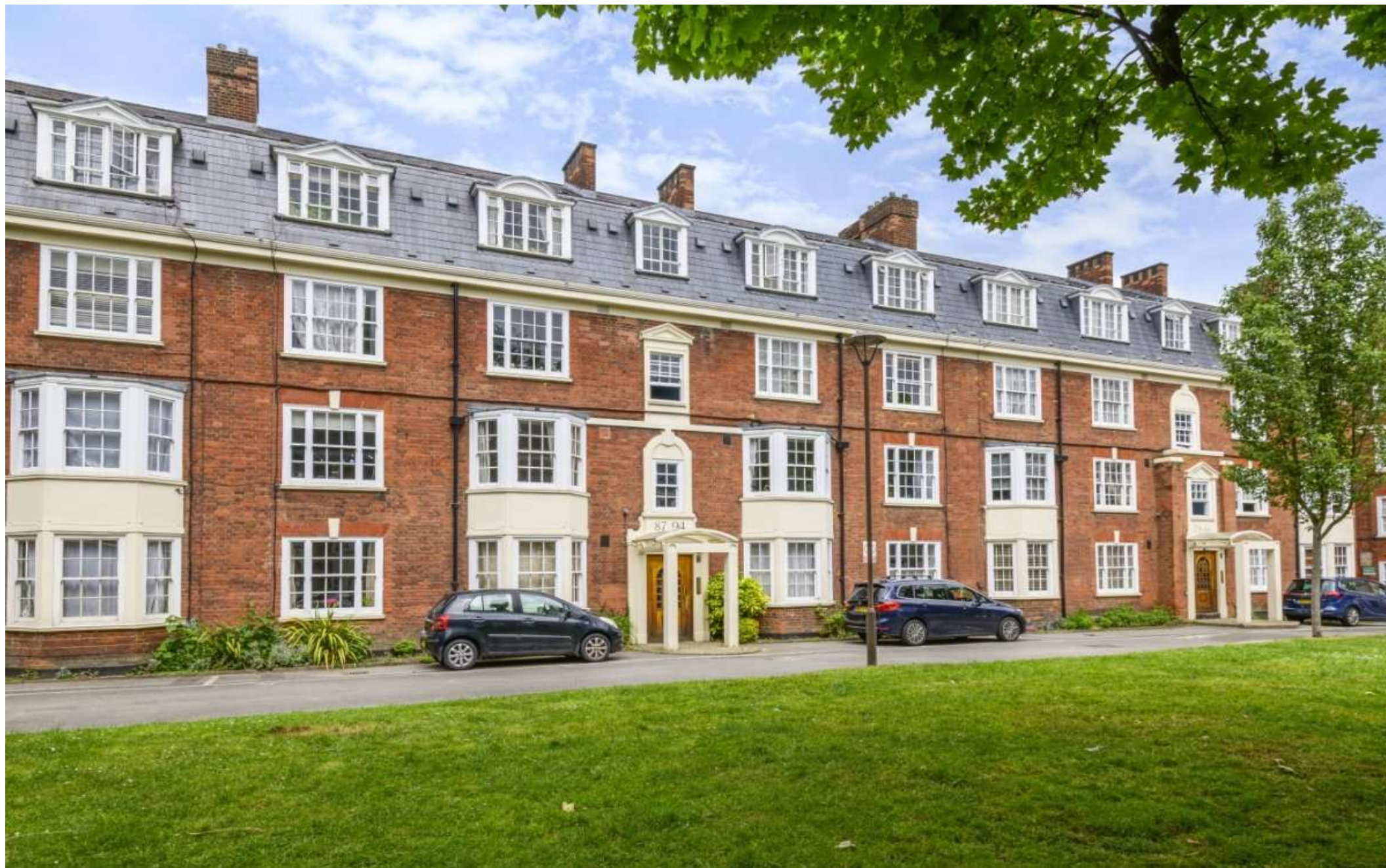
Upper Street, Islington, N1
