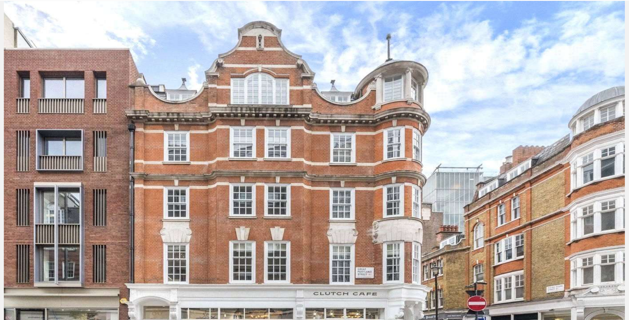
Great Portland Street, London, W1W
