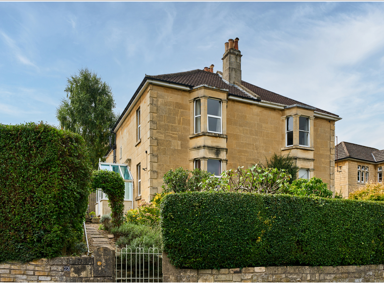
Fairfield Park Road, Bath
