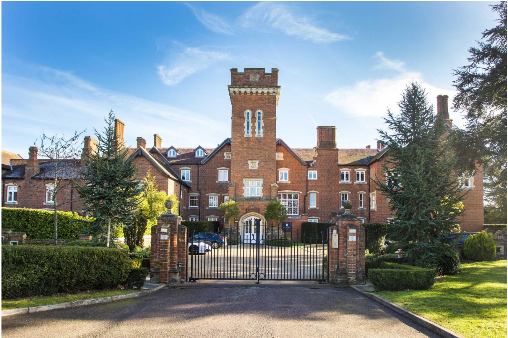
Bedwell Hall Essendon Golf & Country Club AL9
