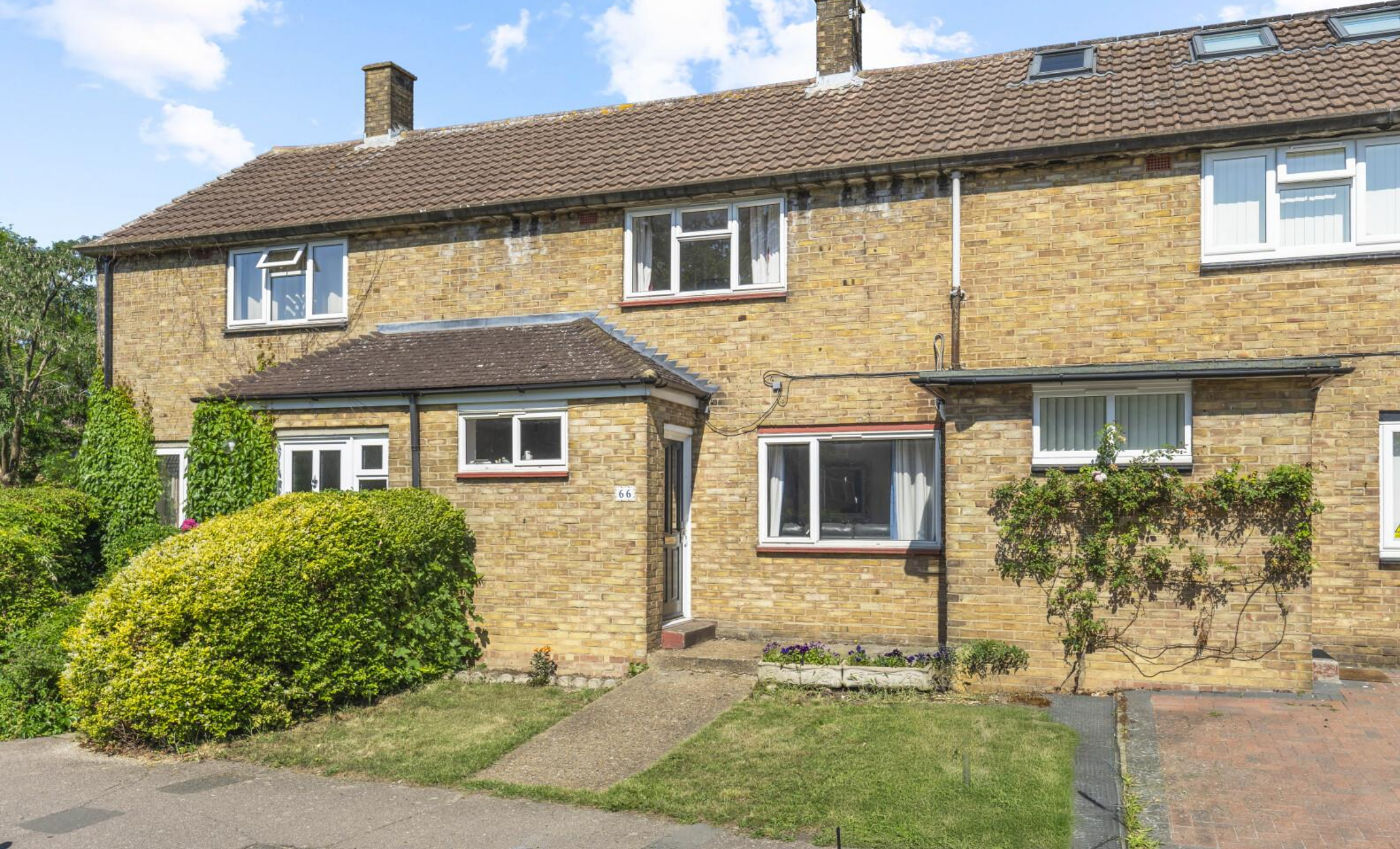
Tunnmeade, Harlow 2 Bedroom House
