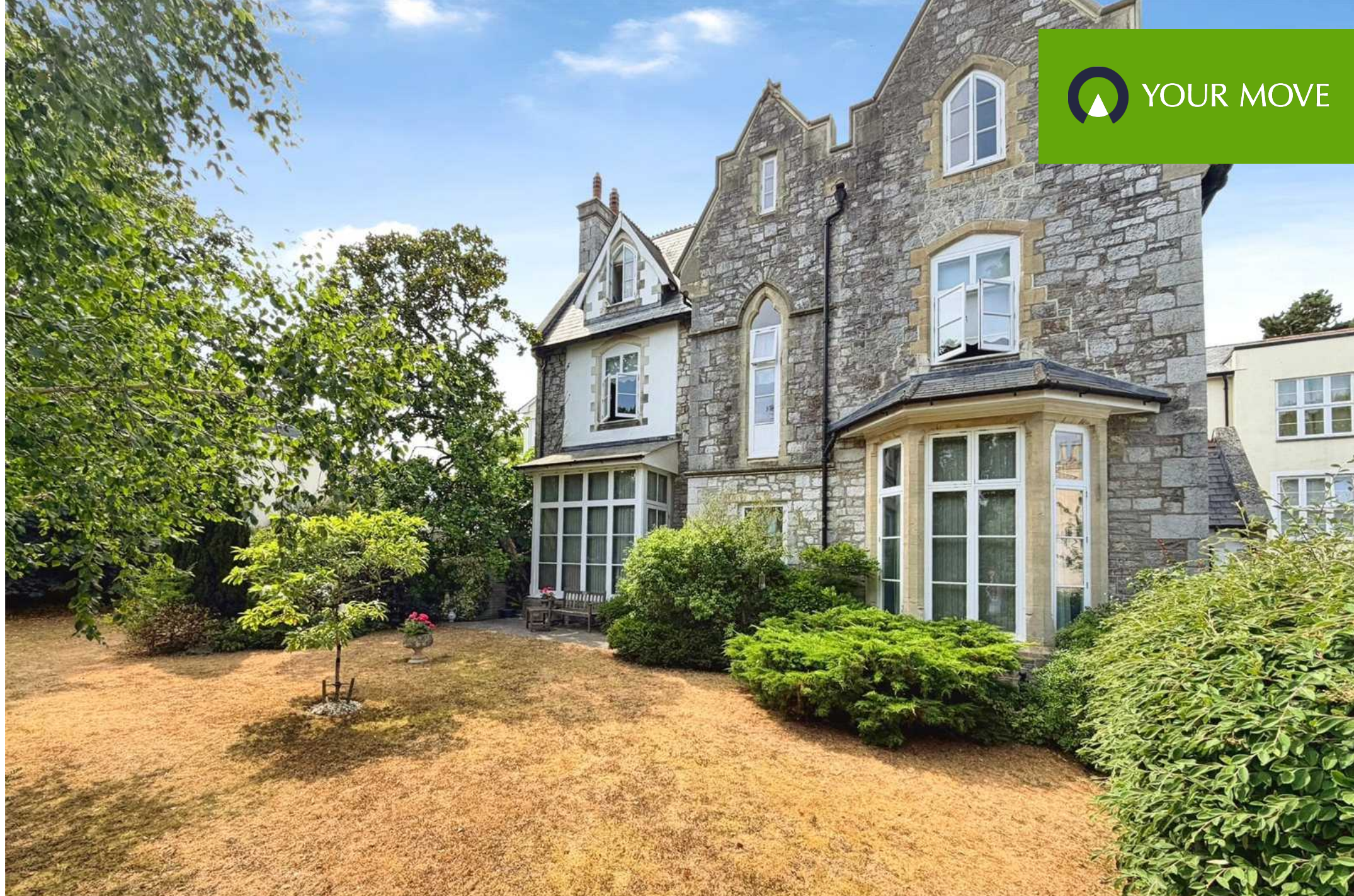
Park House, Courtenay Park Road, Newton Abbot,
