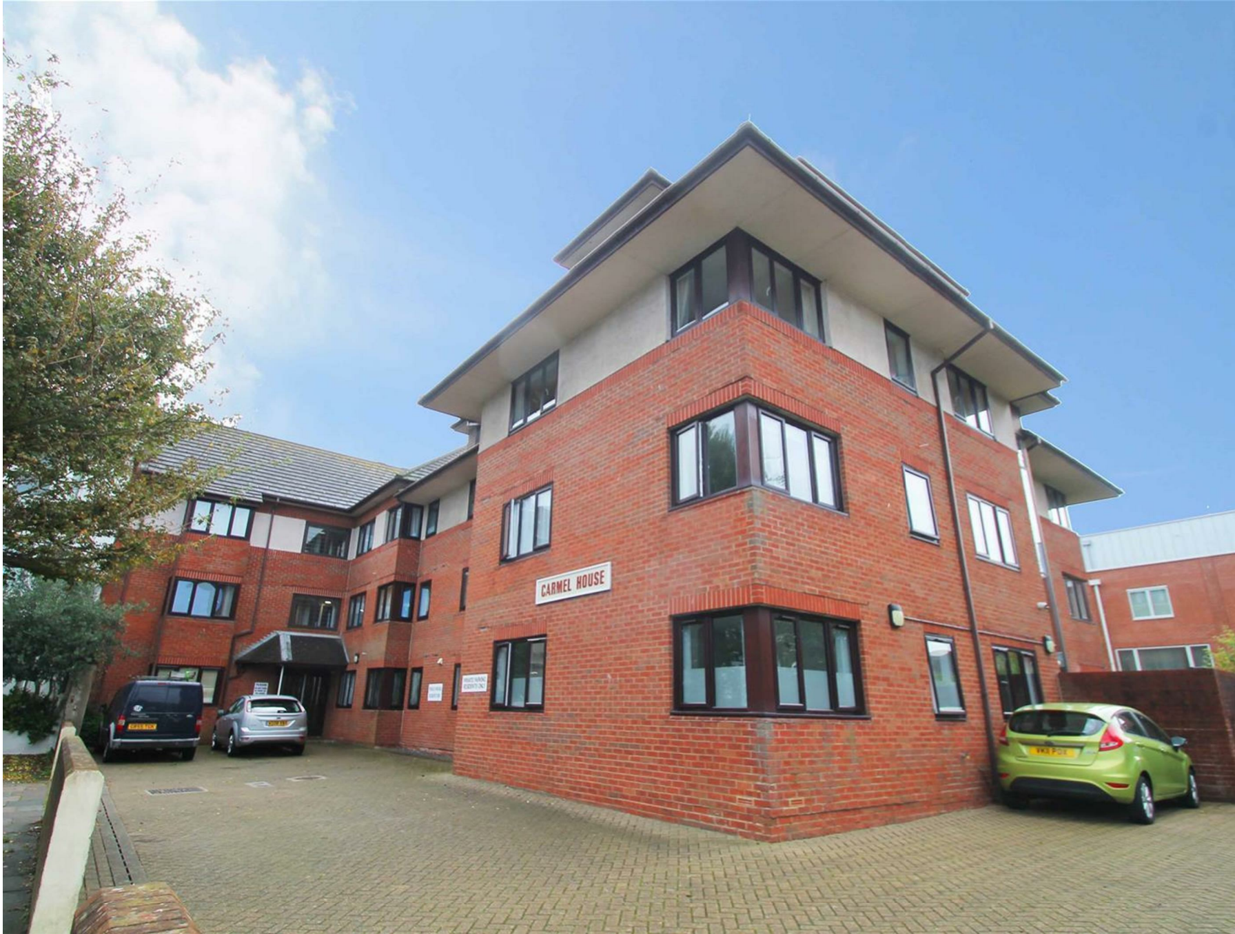
Carmel House, Westbourne Street, Hove, BN3 5PE £150,000 - £160,000 Guide
